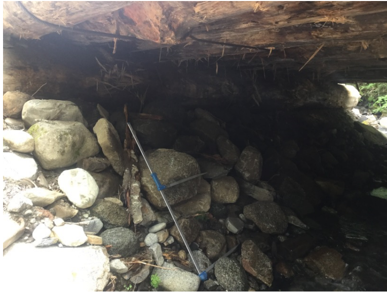
Right Bank Abutment when facing downstream
