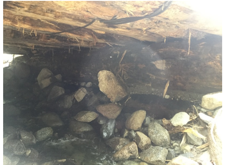
Left Bank Abutment when facing downstream
